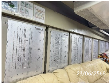
Graphic Annunciator Fire Alarm System
